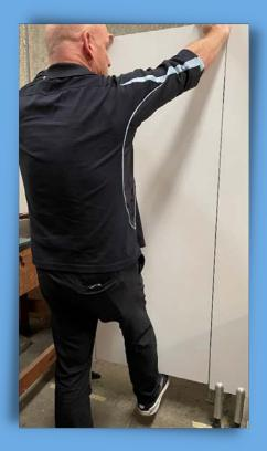
Step 2: Lift the door and when the door clears the hinges and bumper simply turn and move the door towards you and place it next to the cubicle entrance.
